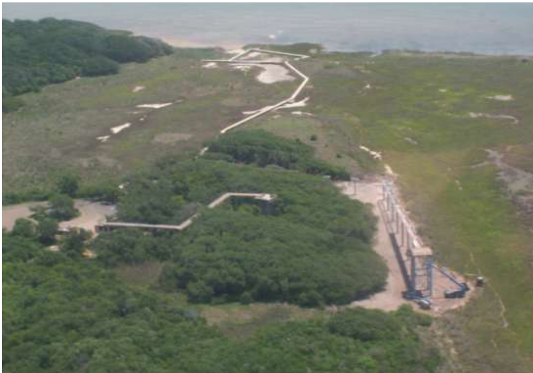
Tower construction built in front of old tower. April, 21, 2009. Photo by Tom Stehn.
