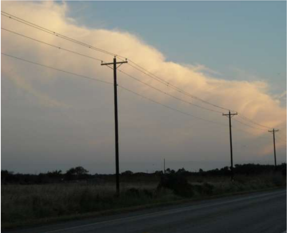
Power line marked by AEP with bird flight diverters on one side of highway by Lamar feeder. October 27, 2010. Photo by Tom Stehn.
